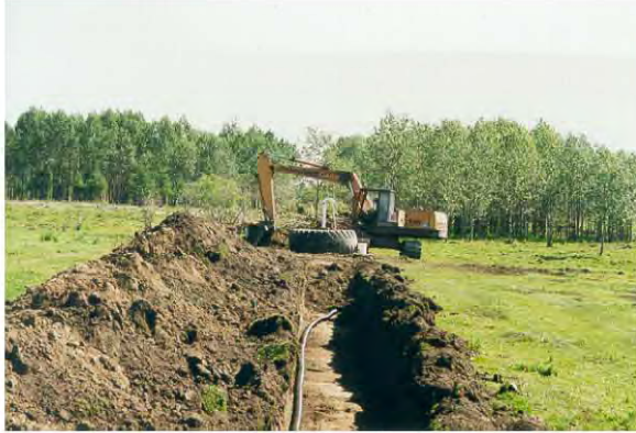
Backfilling the Trenches
